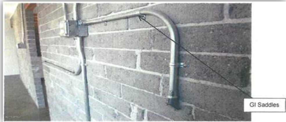
Figure- 25 (Sample Picture) GI Conduit Fixing
