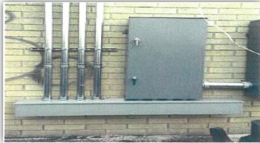
Figure- 26 (Sample Picture) GI Conduit Fixing
