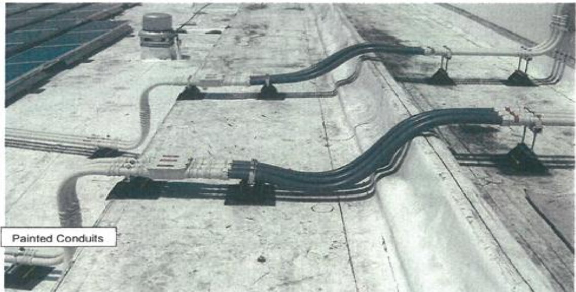
Figure- 30 (Sample Picture) GI Conduits installation at building expansion joints
