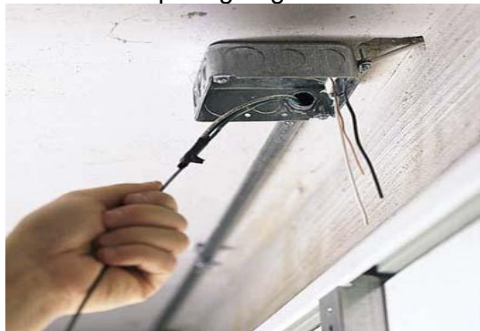
Figure – 9 (Sample Picture) Using Steel Draw Wire for Cable Pulling
