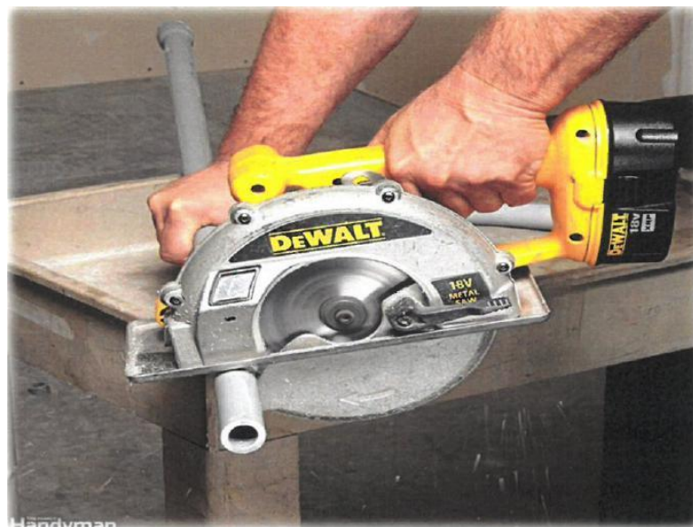
Figure — 3A (Sample Picture) Conduit Cutting Method
